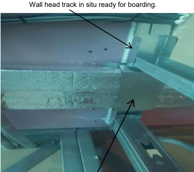
Metal intumescent fire sleeve in situ ready for boarding.
